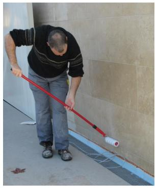
META CRÈME™ was used to seal the pool surround. META CRÈME™ is an ultra-low VOC sealer. The innovative technology creates a deep water-repellent barrier, significantly reducing the formation of efflorescence. META CRÈME™ is invisible, so the travertine pavers will retain their natural color. The wet-slip resistance of the pool surround will also be unaffected.
